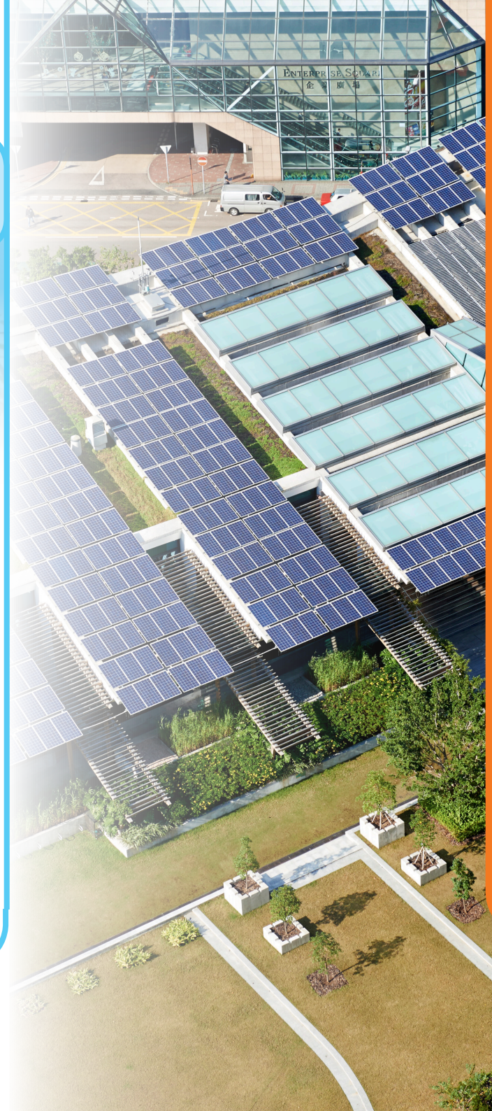
Figure 3.3.1 Photovoltaic panels installed on roof (Source: Hong Kong Science and Technology Park Corporation)
